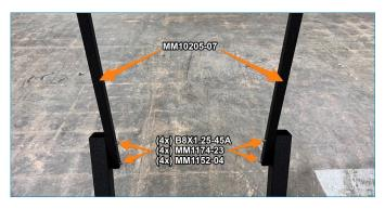
**9.** Use a bubble level to adjust the upper mounts then tighten the (4x) bolts from the previous step (5mm hex key).
